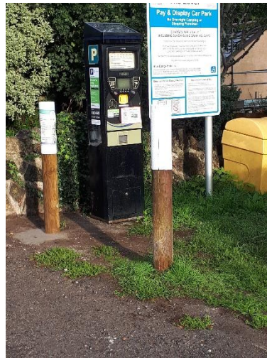
Post replaced and both posts painted white Sept 2026
