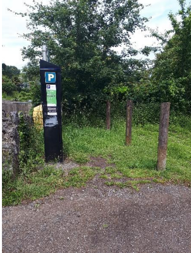
Replacement post required to protect the pay and display machine. June 2026
